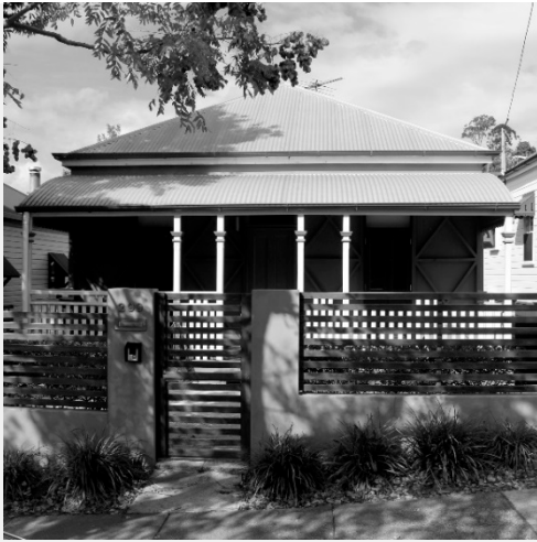
Figure 5-4 Queenslander—tin & timber structure
