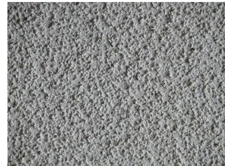
“Popcorn ceiling” with acoustical spray 10
