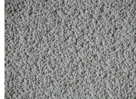
"Popcorn ceiling" with acoustical spray 10
