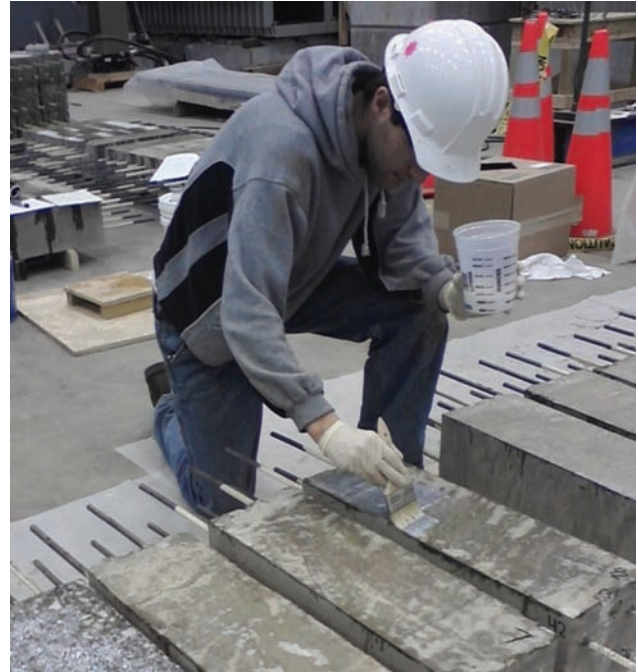
Figure 4.32 Application of Enviroseal 40.
