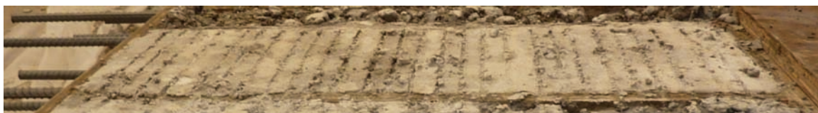
Figure 4.13 Modified shallow tine marks.
