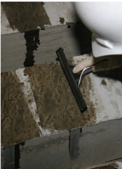
Figure 4.31 Squeegee used to pond product over crack.
