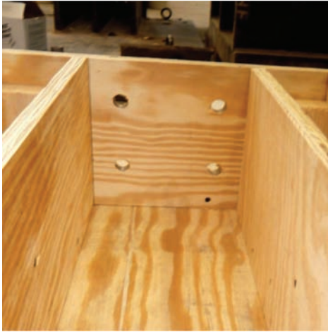
Figure 4.16 Holes for placement of reinforcing steel.
