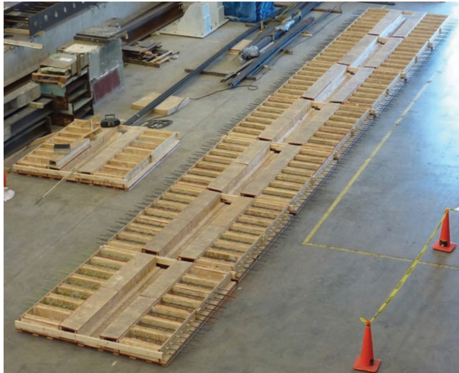
Figure 4.18 Formwork with specimen reinforcement.
