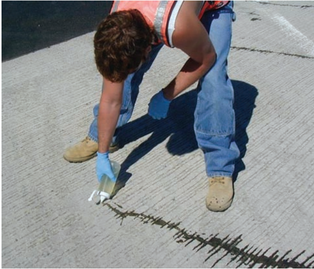
Figure 1.8 Applying a prestripe of crack filler/sealer material (Frosch et al., 2010).
