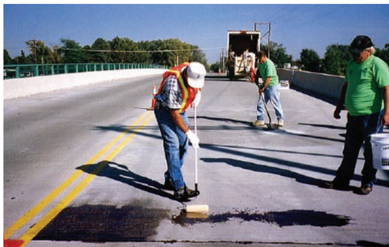
Figure 1.6 Placement of gravity feed crack filler/sealer (Soriano, 2002).
