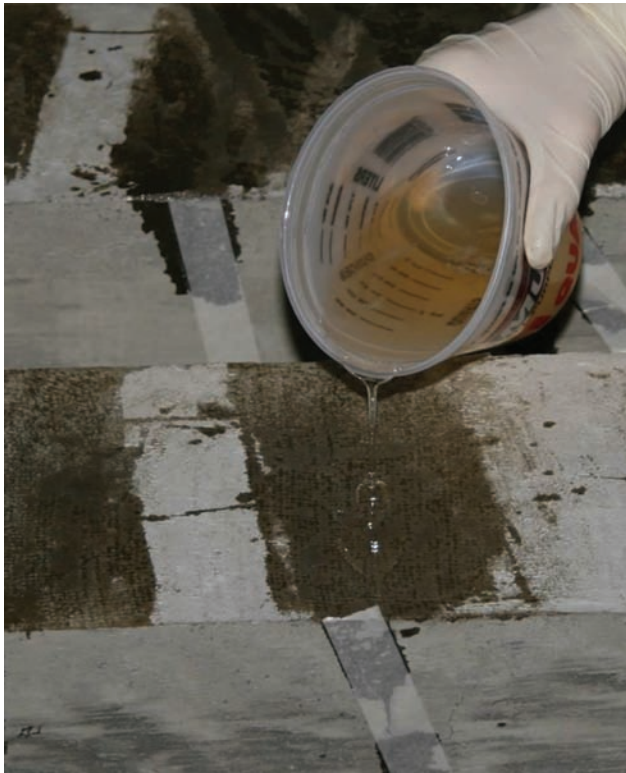
Figure 4.30 Pouring of Sikadur 55 SLV.
