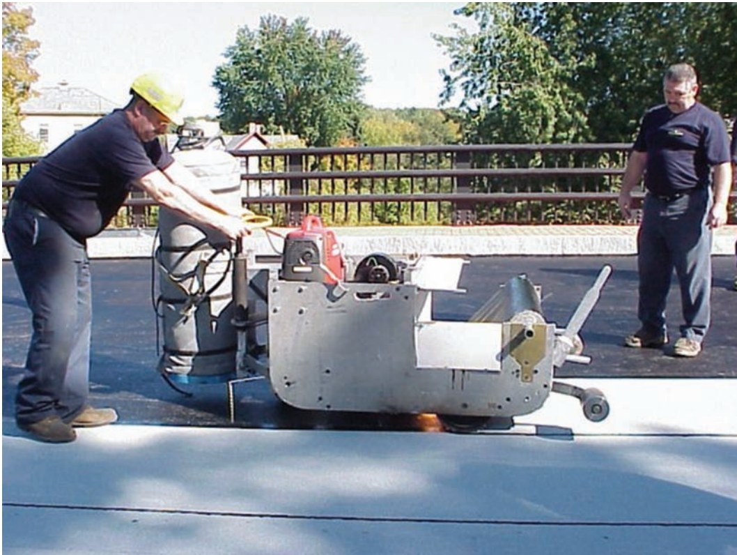
Figure A.12 Small Soprema machine.
