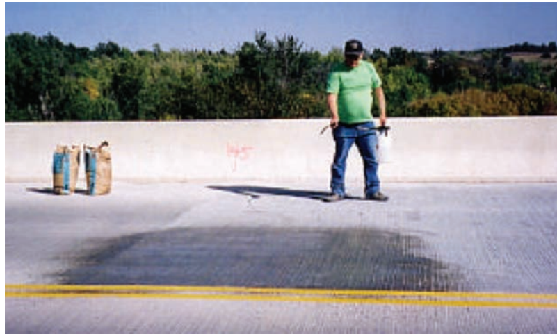
Figure 1.7 Application of surface sealer (Soriano, 2002).
