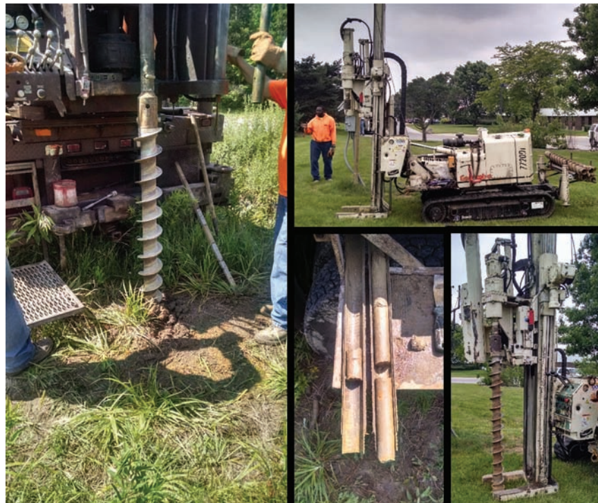
Figure 4.4 Collection of undisturbed soils by drilling rig.
