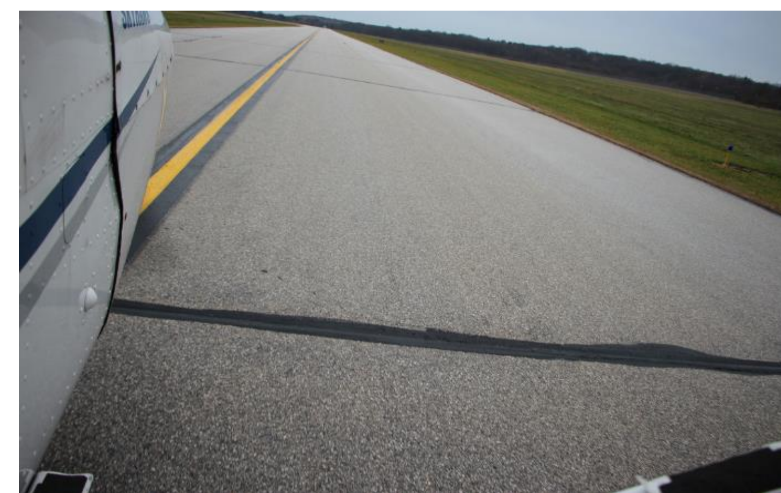
Examples of Transverse Joints from C2 to C3 on Taxiway C at KLAJF
