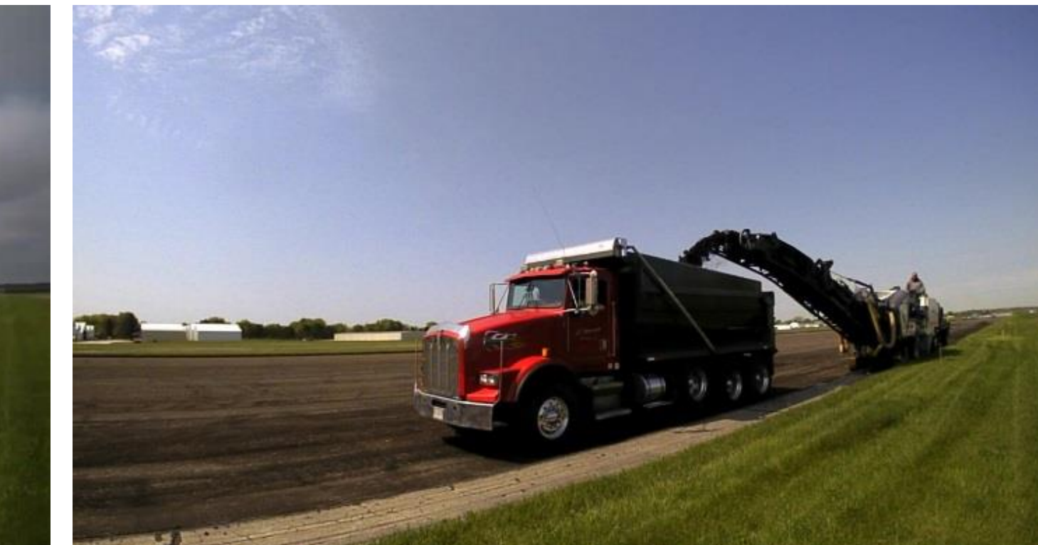
(b) May 6, 10:35 - Milling nears completion
