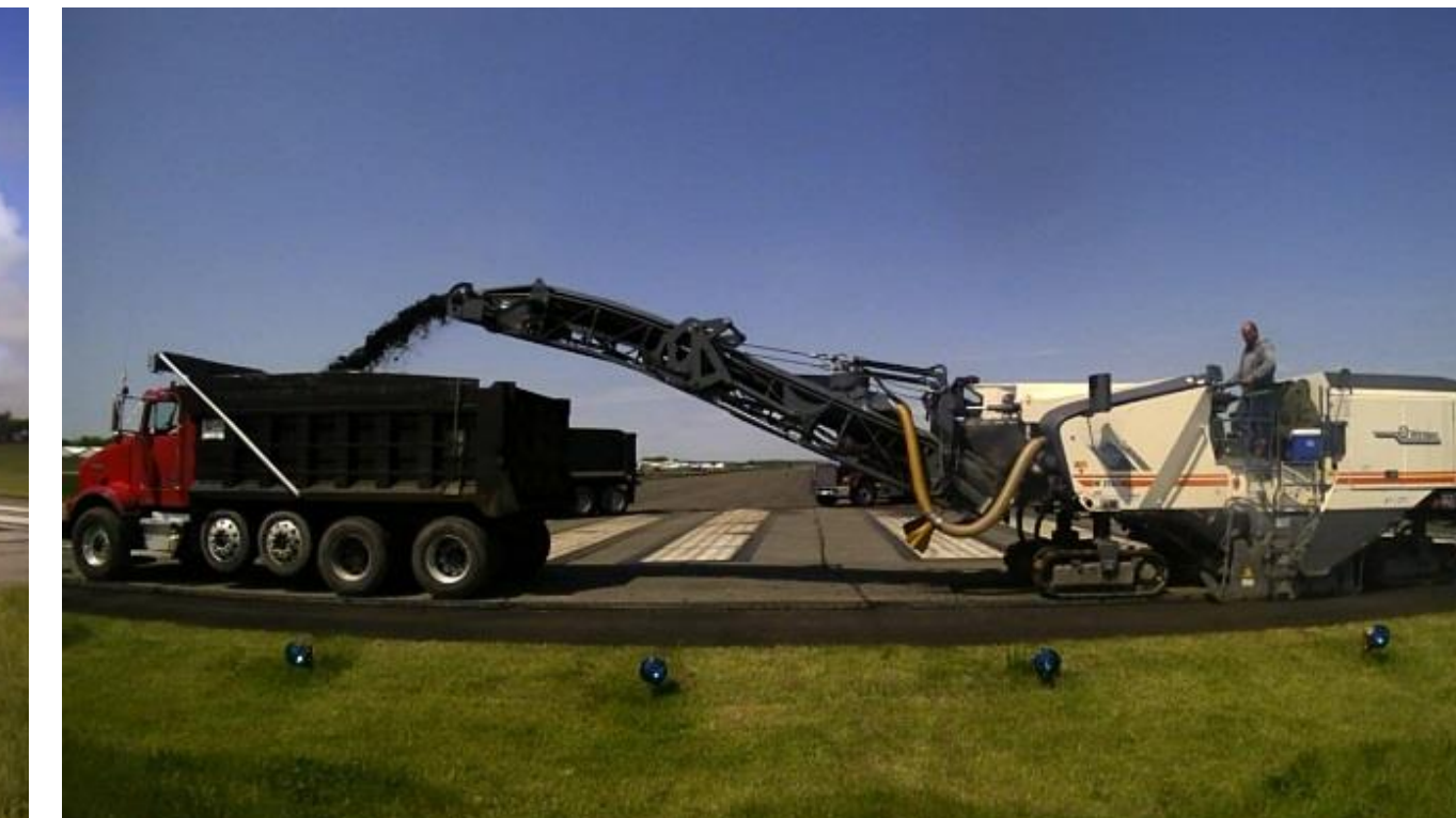
(b) May 6, 11:10 - Milling runway threshold
