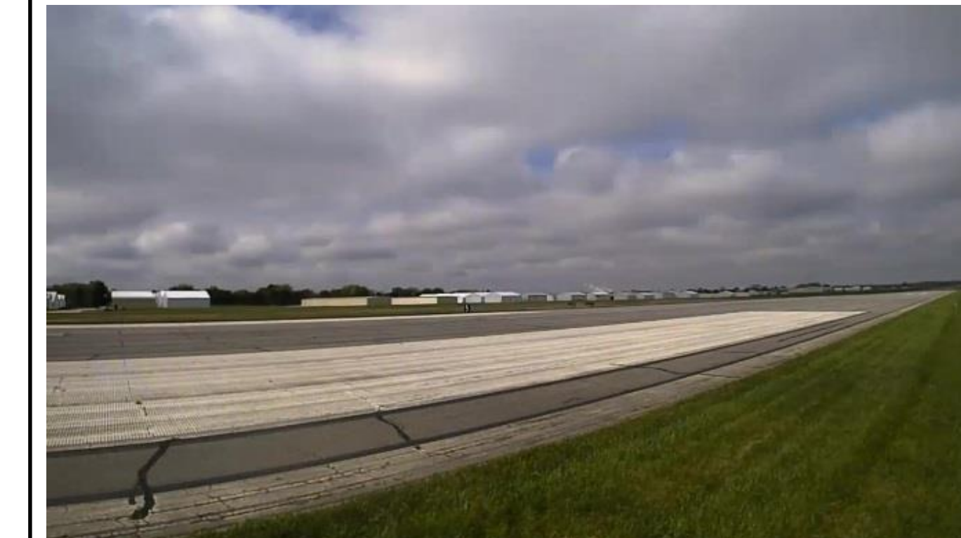
(a) April 29, 11:00 - Original pavement
