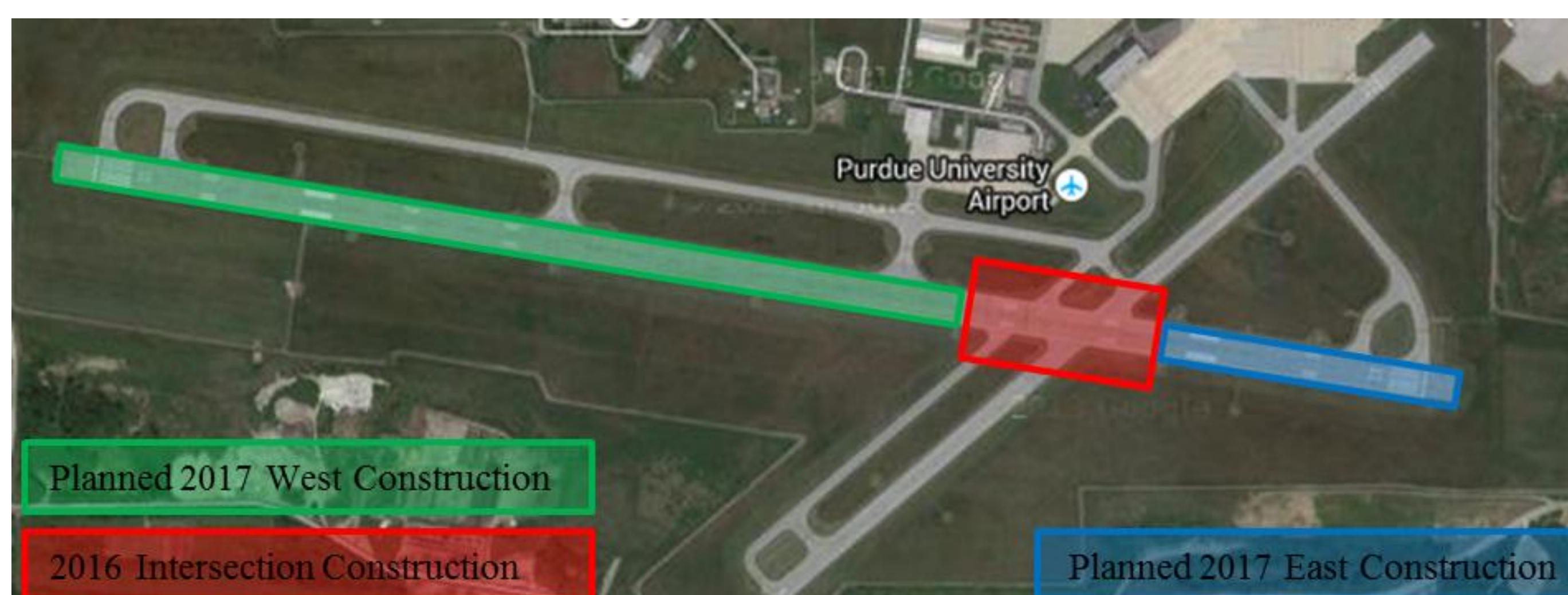
Purdue University Airport (LAF) construction areas
