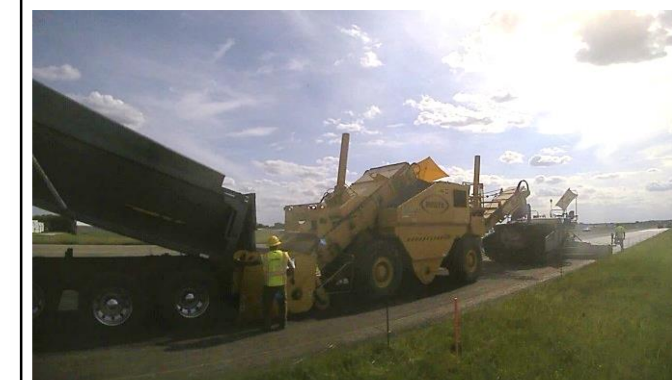
(e) May 25, 16:30 - Asphalt placement started
