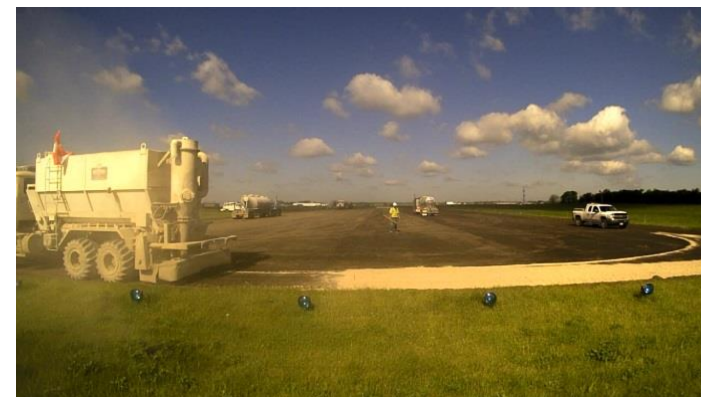
(c) May 13, 09:15 - Soil treatment placed
