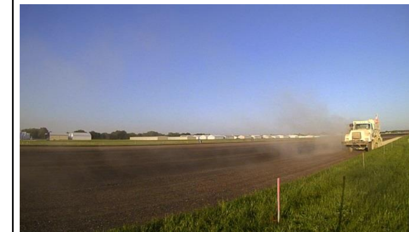
(c) May 13, 07:00 - Soil treatment placed
