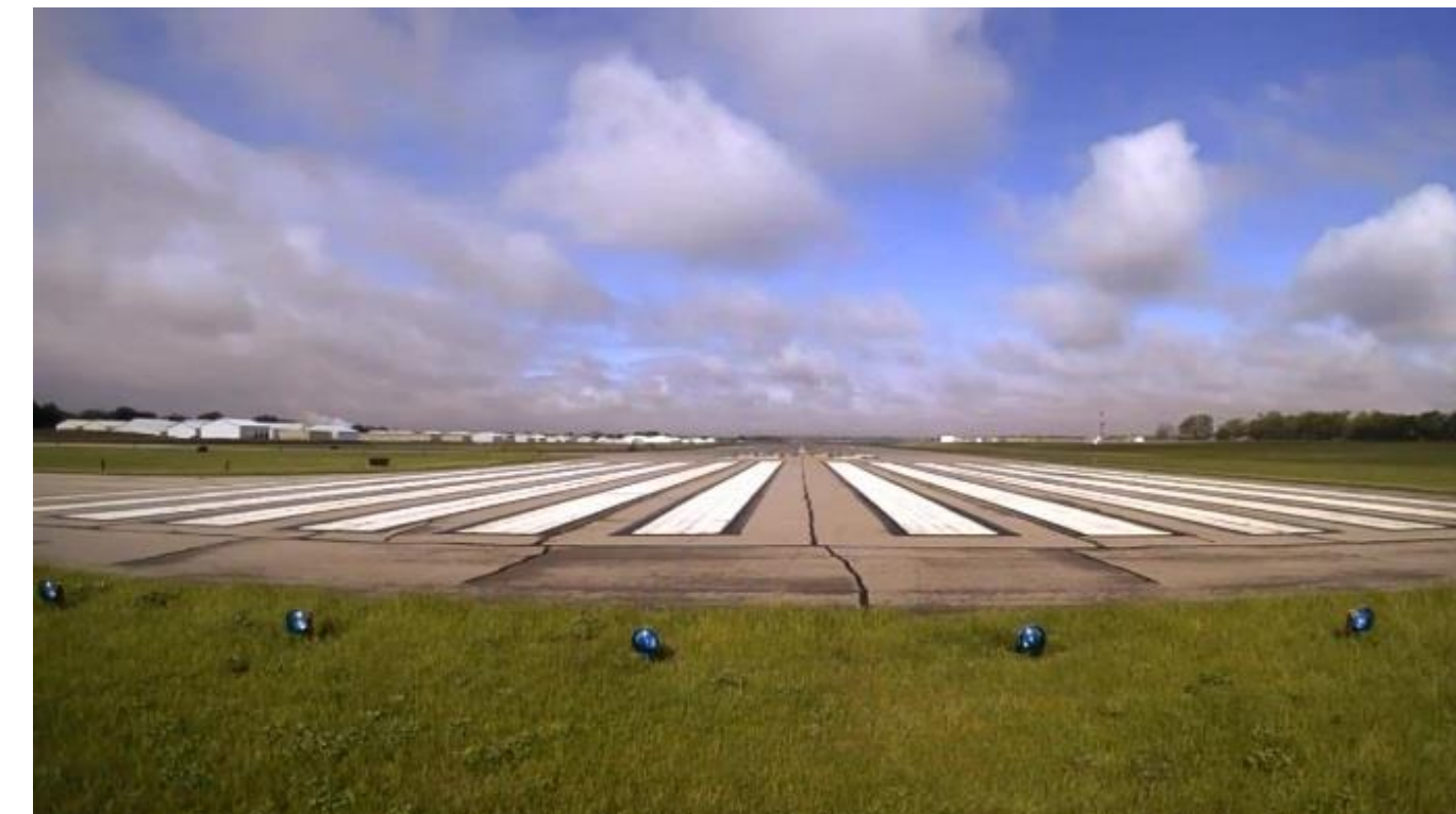
(a) April 29, 11:00 - Original pavement
