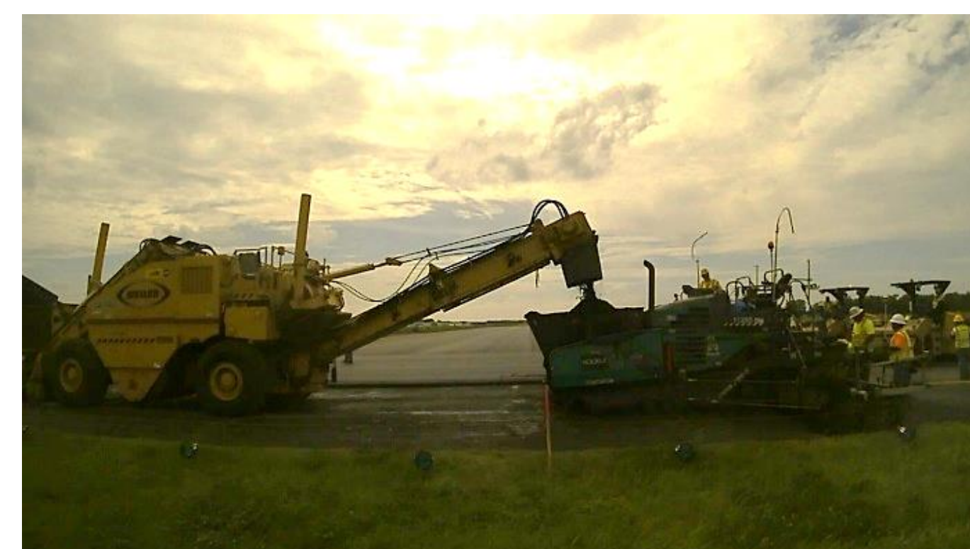
(e) May 28, 15:30 - Asphalt placement
