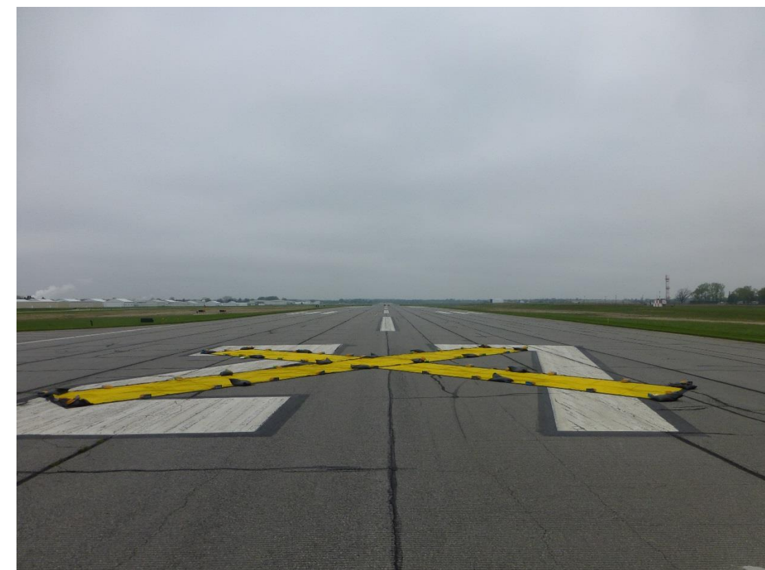
Lights and tarped 'X' for R/W 9/27 closure
