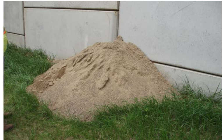
Backfill Leakage
