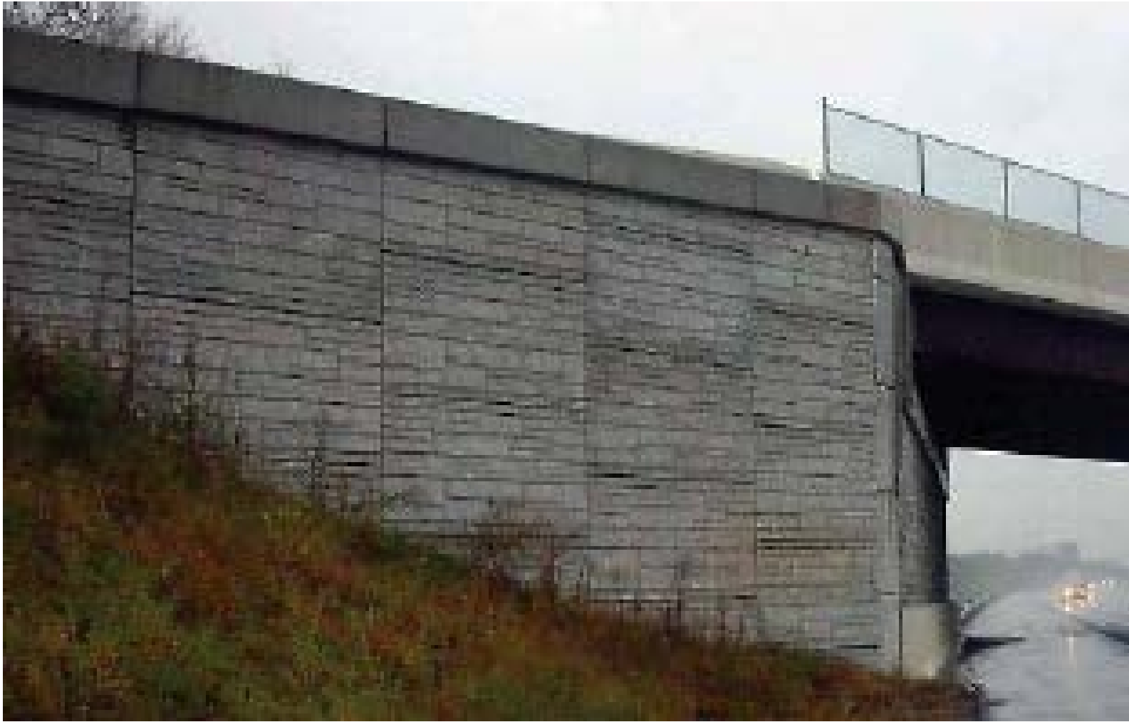
Indiana Toll Road Improvement in Gary
