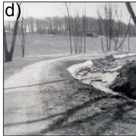
Figure 4.1: Evidence of early bank armouring and reconstructing. a) construction in Edwards Gardens; b) retaining wall in Edwards Garden July, 1961; c) hardening of the left bank looking upstream; d) hardening of the left bank looking downstream. Each were taken in the early 1960s however the exact dates are not known (Toronto Archives, 1961).
