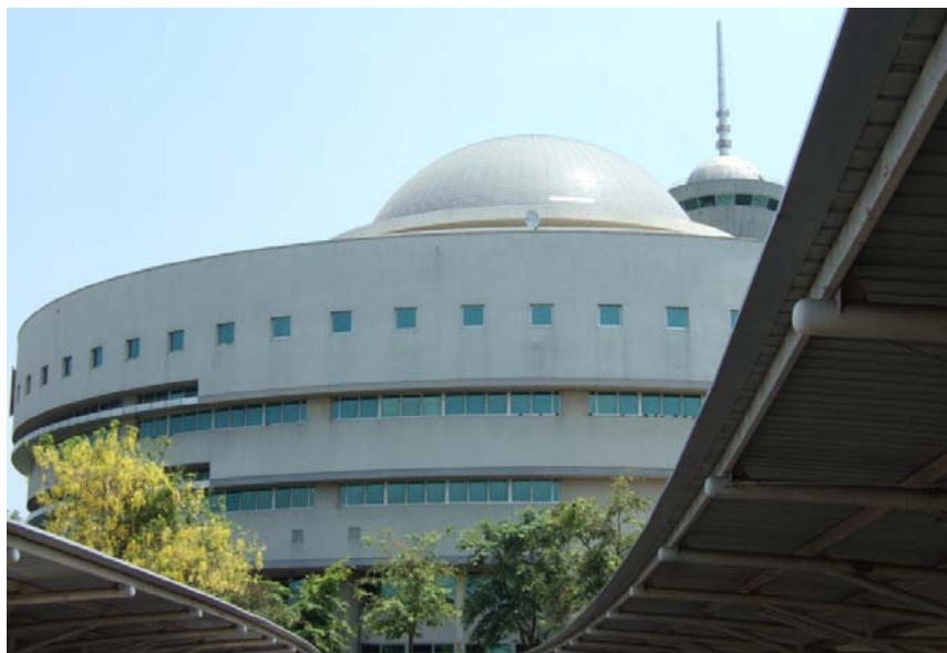
Figure 24 – The award-winning building of Shinawatra University, Sam Khok district, Pathumthani province, Thailand. © 2014 Photo by B. R. Buergi.
