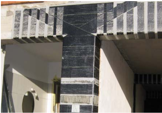
(a) EB-FRP strengthening of beams
