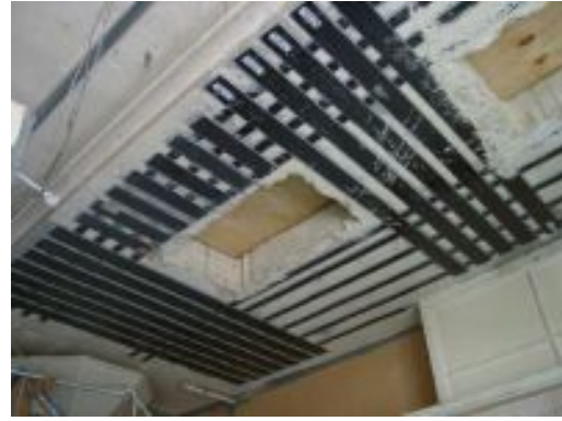
(b) EB-FRP strengthening of slabs
