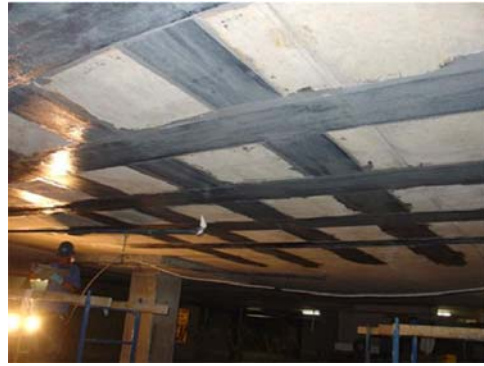
(b) Leon county courthouse parking garage-2
