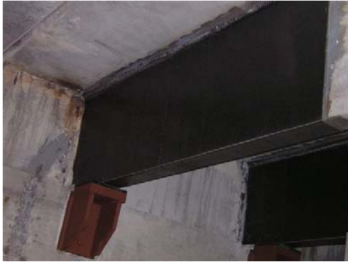
(a) EB-FRP strengthening of beams
