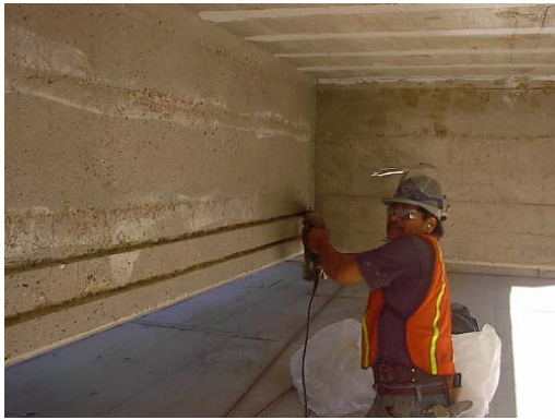
(e) NSM-FRP strengthening of beams
