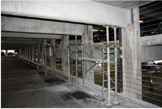
(a) Leon county courthouse parking garage-1
