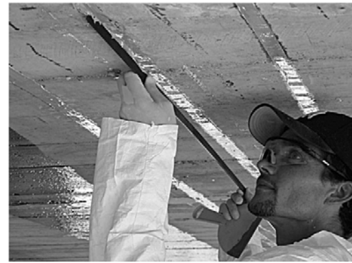
(f) NSM-FRP strengthening of slabs
