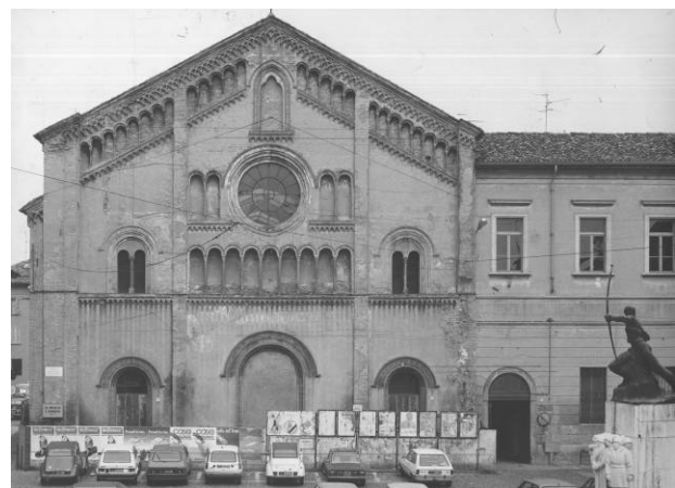
Figure 1: Church of San Domenico in Crema (Cr) 1984. The rectified image has been taken directly photographically with a reflex camera with a tilt-shift lens and later plotted at 1:50 scale. (Degree Thesis, Campanella Zucchetti)
