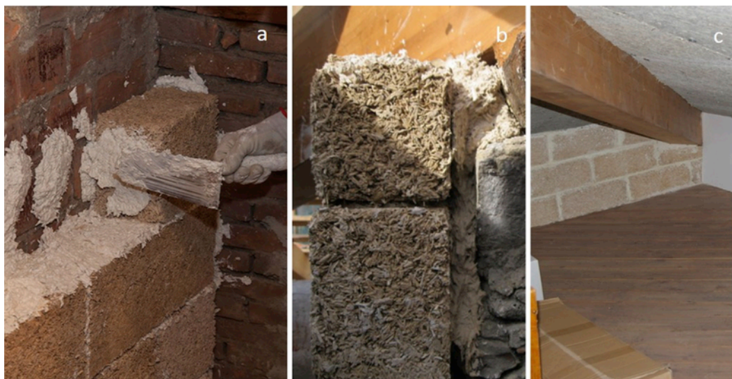
Fig. 1. Details of non-load-bearing walls made of hempcrete blocks: (a) wall erection; (b) side view; (c) front view.
