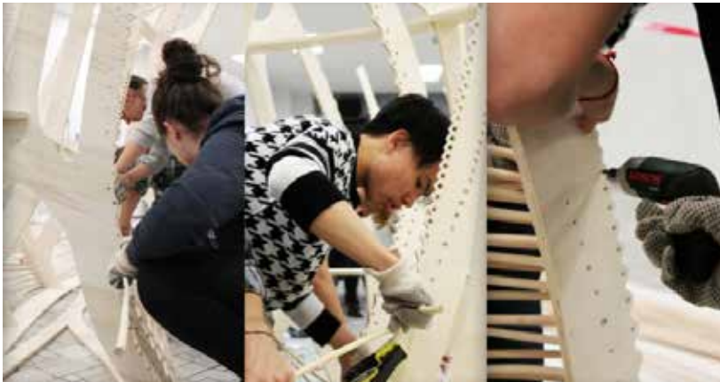
Figure 16: Manual work is still a fundamental step in the weaving process. Right. Screwing process for rattan post-tensioning
