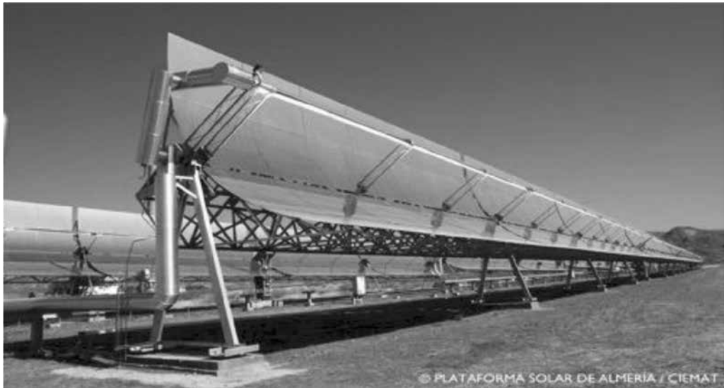
Figure 8: CSP trough at Plataforma Solar de Almería, Spain
