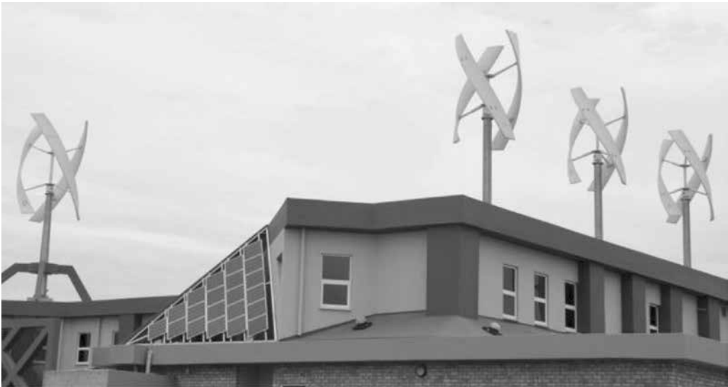
Figure 10: Vertical axis generators in conjunction with photovoltaic seen in Swakopmund Photo: Amusha (2015).
