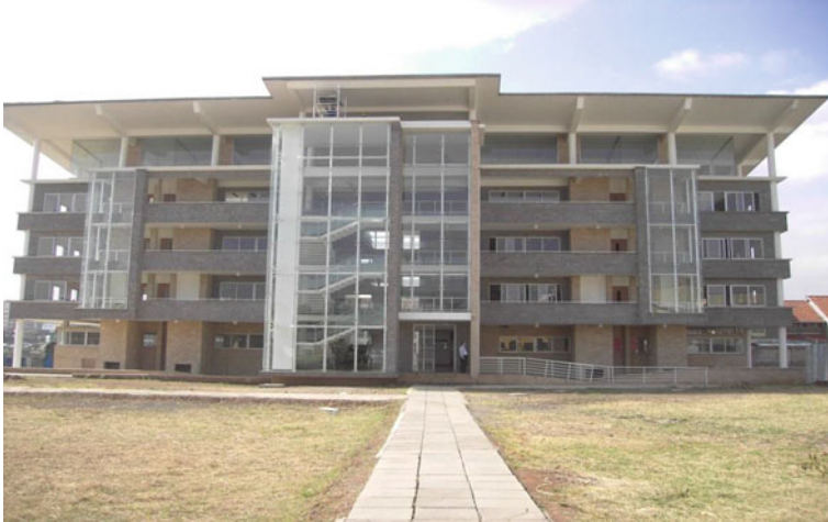
Fig. 1 Management science building at Strathmore University
