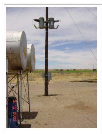
32kVA in parallel to a 48 kVA transformer – irrigation project, 3 phase submersible pump powered via a 11kVA converter drive
