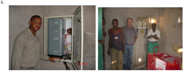
15 kVA converter drive for a 1ton/hour throughput 15kVA motor driven hammer mill. Large single phase motors (up to 22kW available) but have only been used extremely successfully for 7.5KVA applications – to drive mono pumps and pumping water from up to 180m. Standard 3.7 kVA 1 phase motors (460V) are connected to drive deep well pumps.
