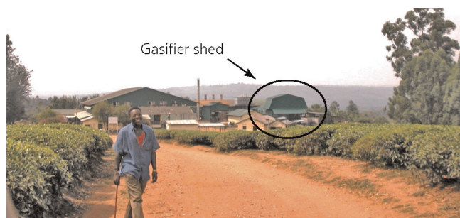
Figure 1. Muzizi Tea Estate processing facility with gasifier shed
