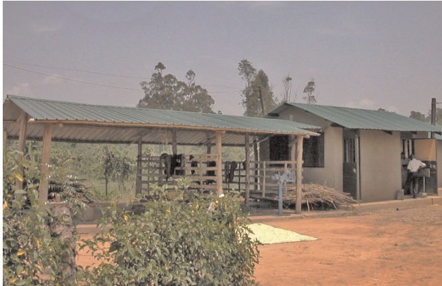
Figure 7. Gasifier shed with fuelwood storage and processing shed attached
