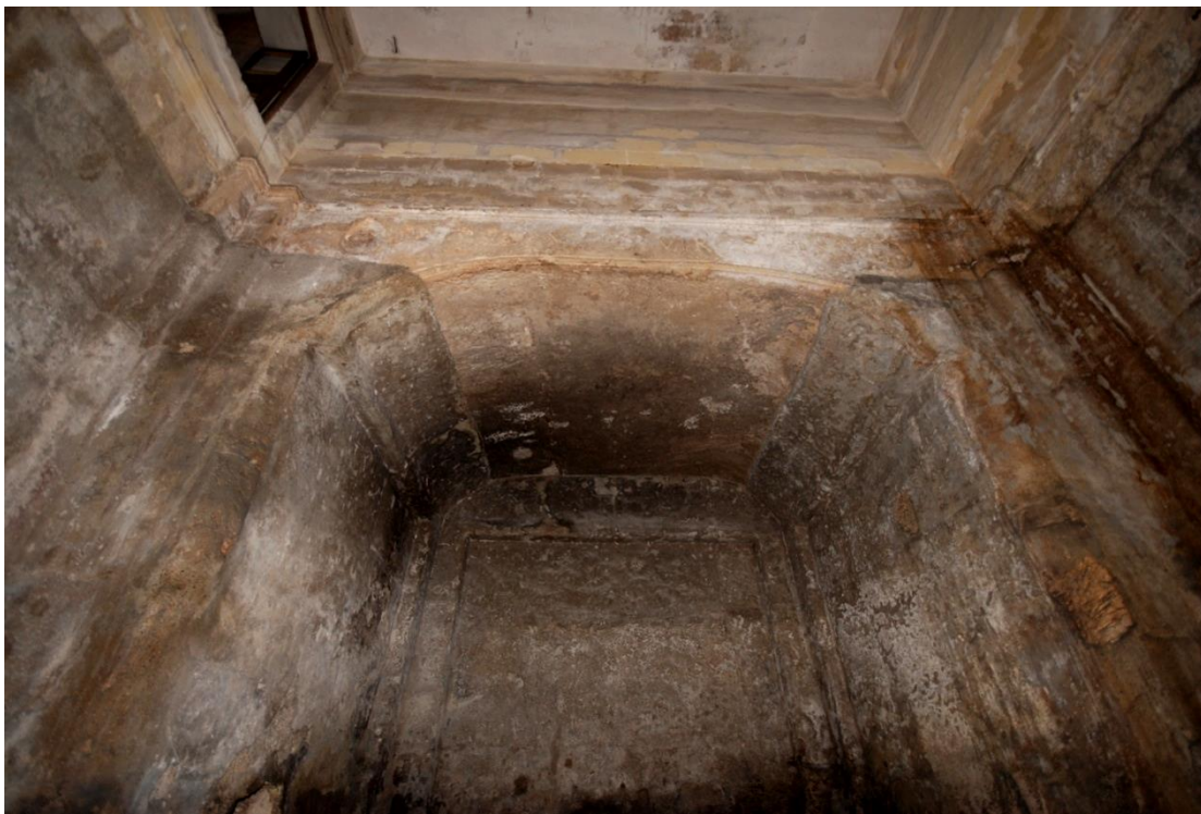
Perspective view of the main apse of the rock-cut church at Bormla. The courses above were added after its rediscovery in 1946. © Photo: Author.
