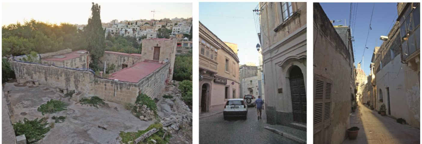
Figure 1. Ir-Razzett tal-Hursun, an original, rural vernacular farmhouse, restored and rehabilitated into the Mediterranean Institute of the University of Malta (left), Main Street, Birkirkara (centre) and Parish Street, Mqabba (right).
