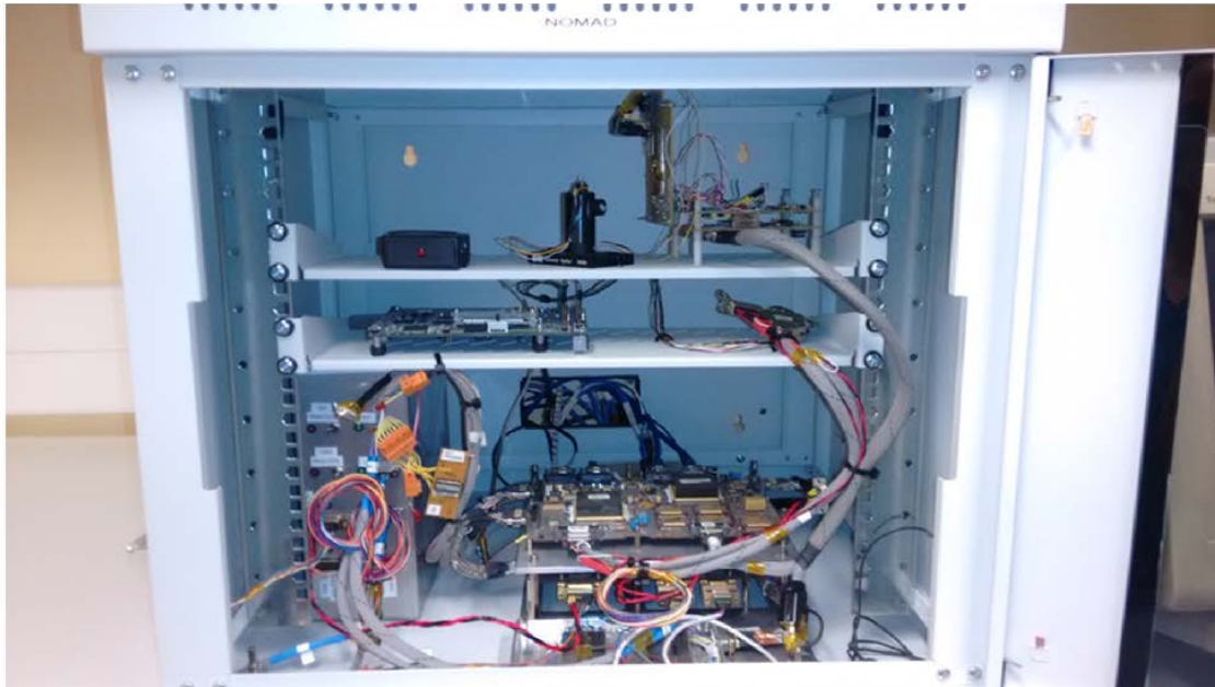
Figure 13 Enclosed EM ready to develop SW
