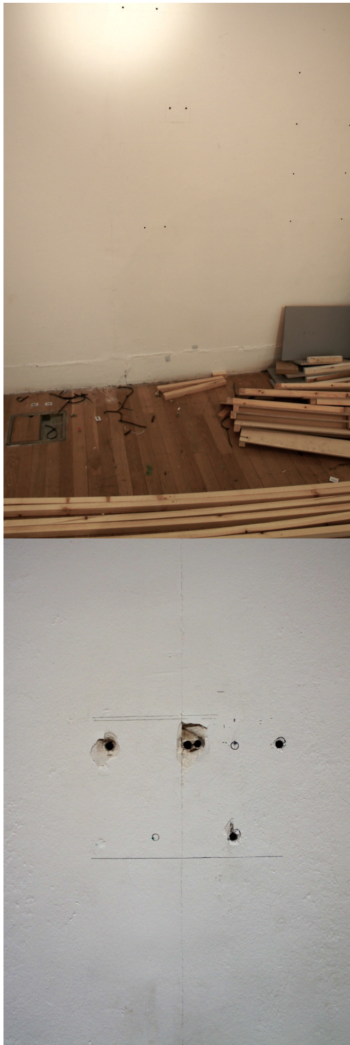
Fig 66. De-installation in Link Gallery
