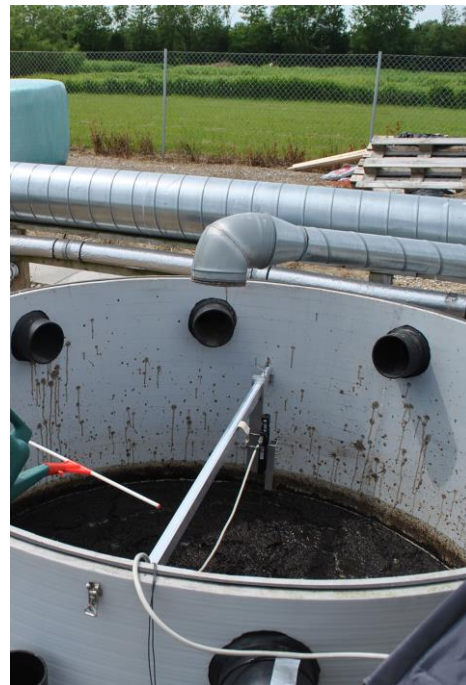
(b). The aluminum bar installed on the inner rim of the slurry tank.
