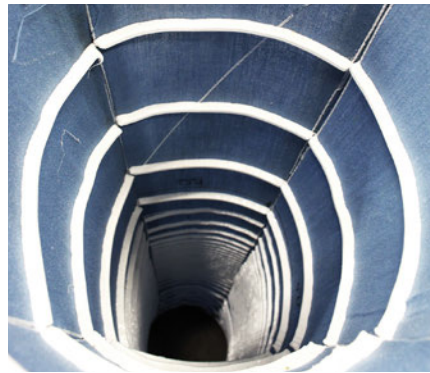
Figure 6. Waisted Column. Manufacturing process, from casting to removing the fabric formwork. Photo: Cristina Nan and Charlie Patterson.
