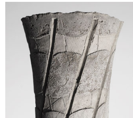
Figure 8. Twisted Column. Manufacturing process, from casting to removing the fabric formwork. Photo: Charlie Patterson.
