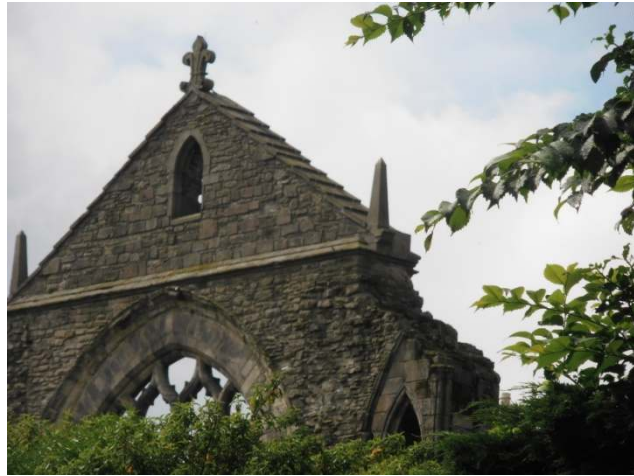
Figure 8. Remains of the Douglas and McPherson project at the rubble stonework blocking the openings of the triforium (item 8 in Table 1) and possibly the coping stones at the W gable window (but not the obelisks and fleur-de-lis finial).
