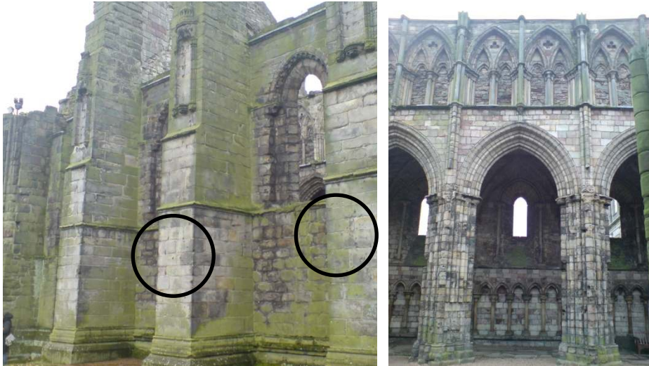
Figure 3. Evidence of gunfire damage at the exterior (from the 1544 invasion) and deep cuts on the shafts of the piers for the insertion of pews at the interior during the extensive refurbishments of 1633 and 1670.
