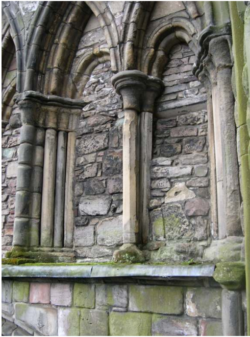
Figure 8. Remains of the Douglas and McPherson project at the rubble stonework blocking the openings of the triforium (item 8 in Table 1) and possibly the coping stones at the W gable window (but not the obelisks and fleur-de-lis finial).
