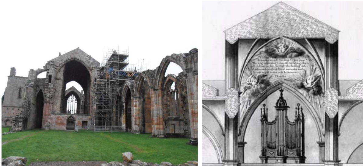
Figure 11. Misinterpretations of vault design in post-reformation Scotland: the barrel vault that replaced the nave cross vaults in Melrose ca 1621 and James Craig's design of the King's Seat in St. Giles, Edinburgh in 1777 (NMR catalogue number C 96508 PO)
