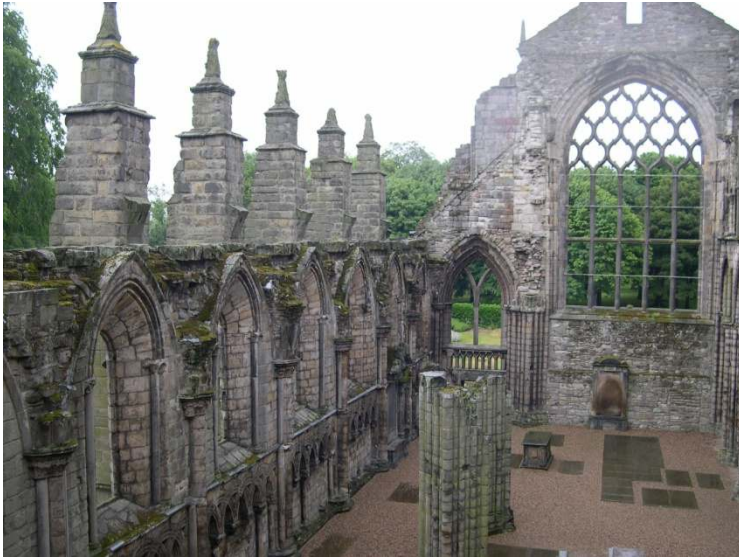
Figure 1. The current state of the abbey church of Holyrood (2010) following no major interventions after the collapse of 1768
