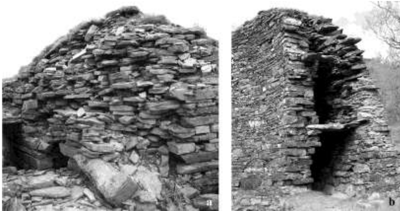
Illus. 3 Different types of broch wall construction: a) well-coursed drystone masonry maintained throughout the wall core (Broch of Borwick, near Yesnaby, Sandwick, Orkney Islands); b) double-wall construction consisting of an inner and outer wall leave interlinked by horizontal lintels (Dun Troddan, Glenelg, Skye and Lochalsh, Highland) (Photographs: T. Romankiewicz)
