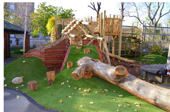
Fig. 1 A new playground construction in the Camden Active Spaces project
