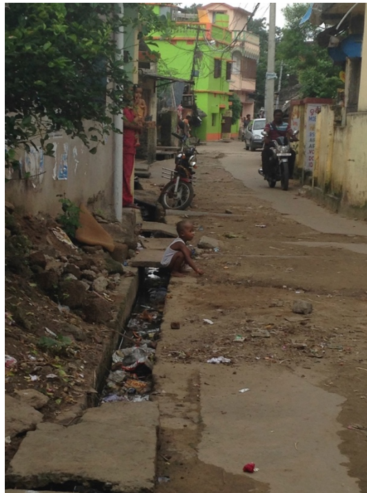
Figure 4.6: Child defecating in a drain
