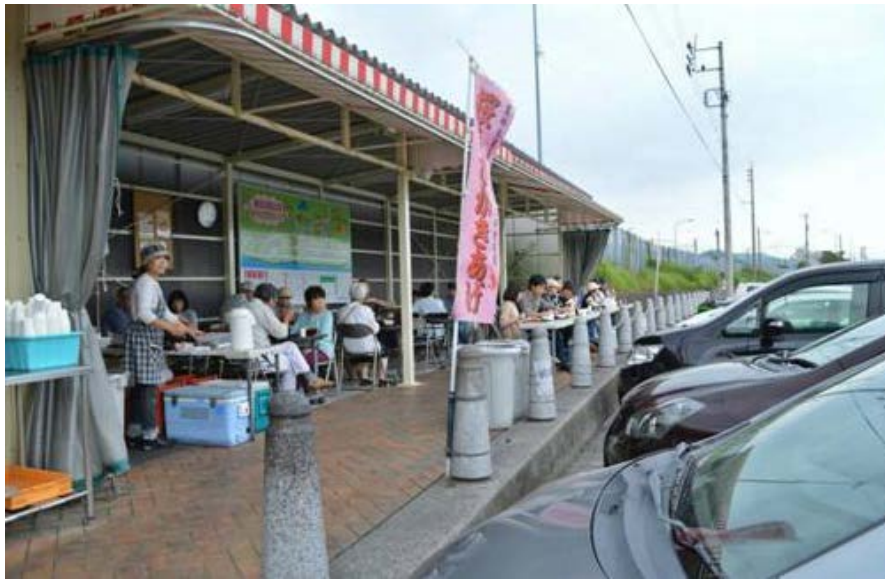
The main building is a very simple construction
