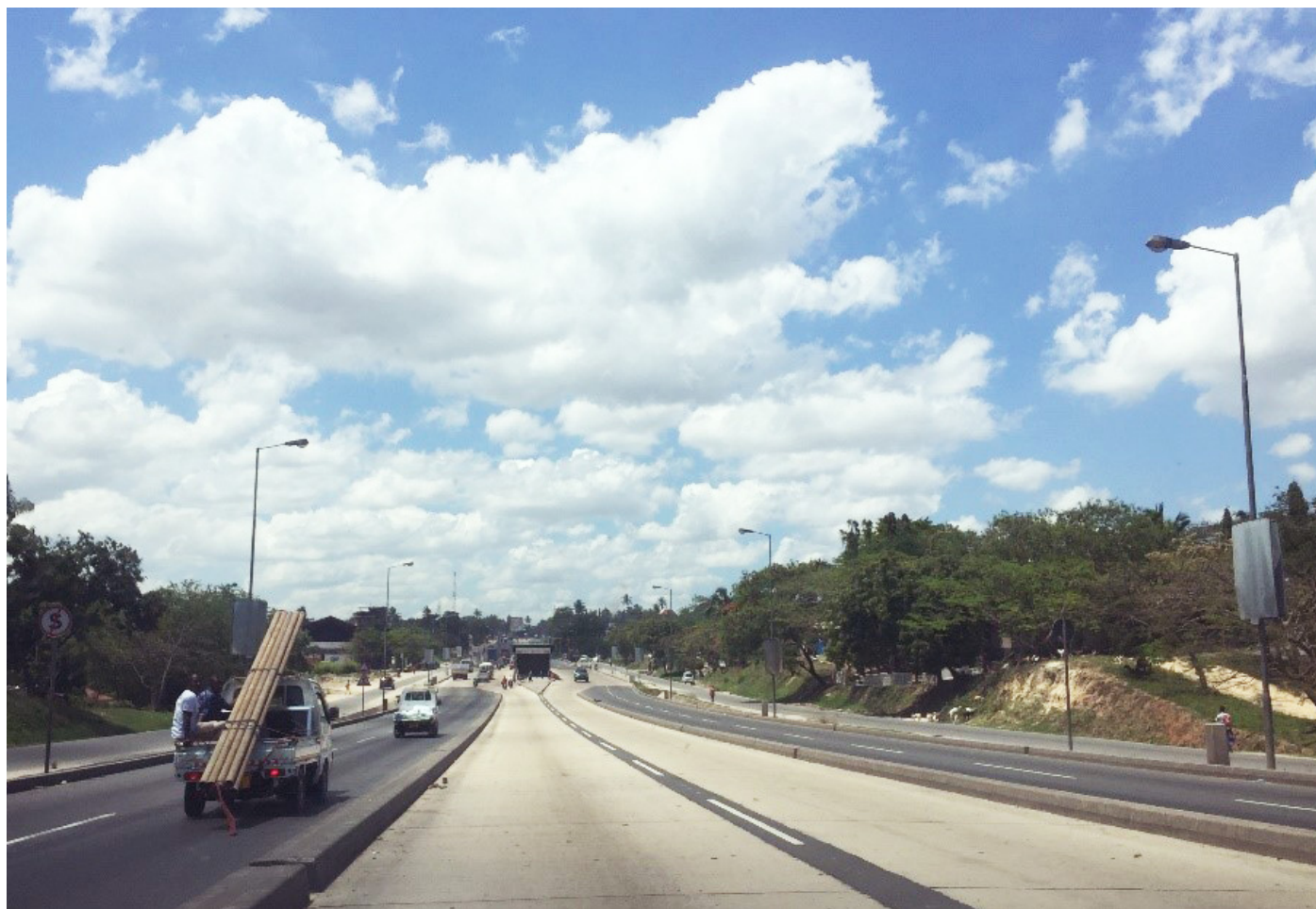
Image 1. Dedicated Bus Rapid Transit (BRT) Lanes in the center of Morogoro Road, Dar es Salaam, Tanzania
