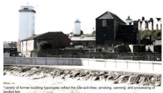
*variety of former building typologies reflect the site activities: smoking, canning, and processing of landed fish
