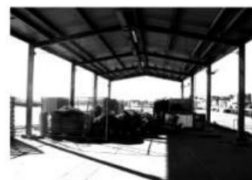
*the fishing industry buildings today with its stripped back, structural fishing sheds providing an industrial backdrop to the site
