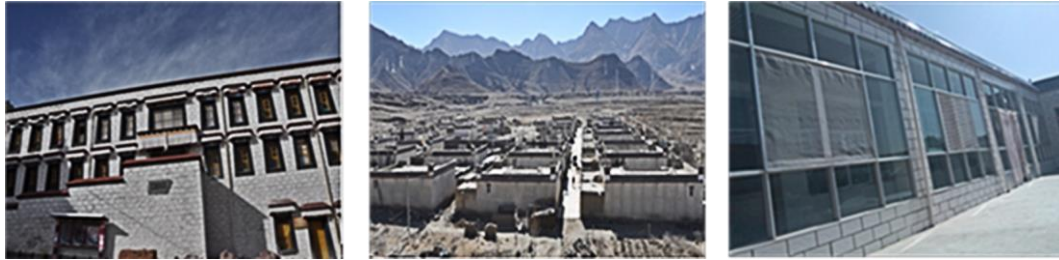
(a) Three-story stone-wall (b) One-story rammed-earth wall (c) One-story solar house
