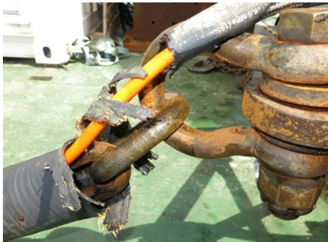
Figure 20: Damage to cable protective hosing at top of sensor frame
