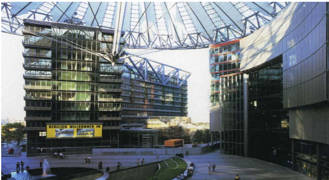
Figure 4: The Forum's roof structure, entrances and central plaza
