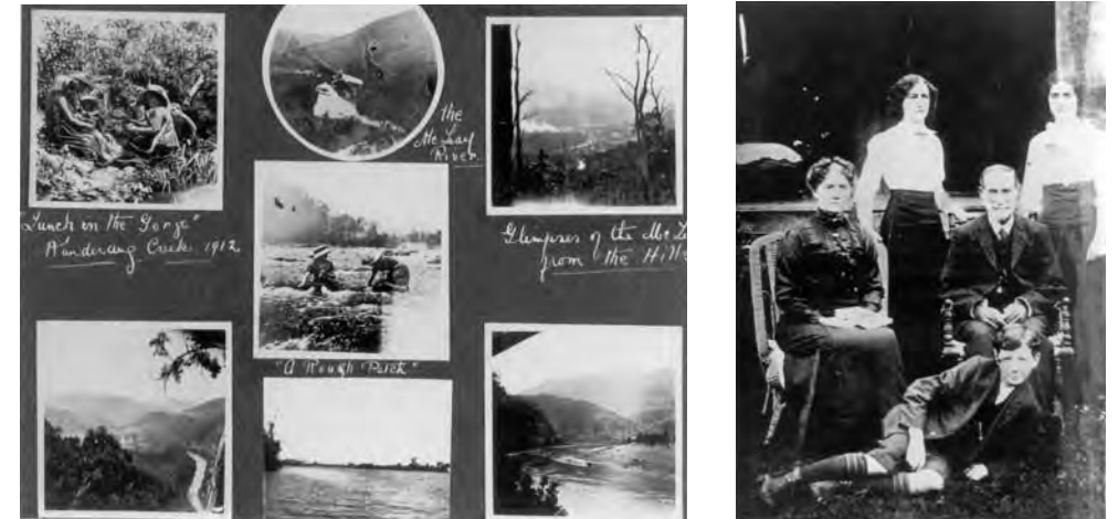
FIGURE 4.12 (left) The Fitzgerald and McDonell Family photograph albums, collected and annotated by Chris Sullivan (1989) provide an invaluable source of documentation for understanding the history of East Kunderang.
