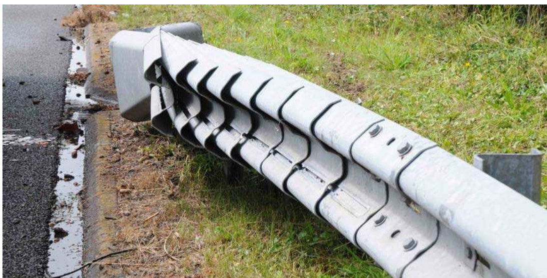
Figure 5.8(ii): Compressed Roadside Barrier [GP]
