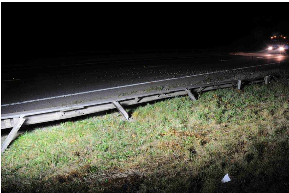
Figure 5.5(vi): View of collapsed roadside barrier [GP]
