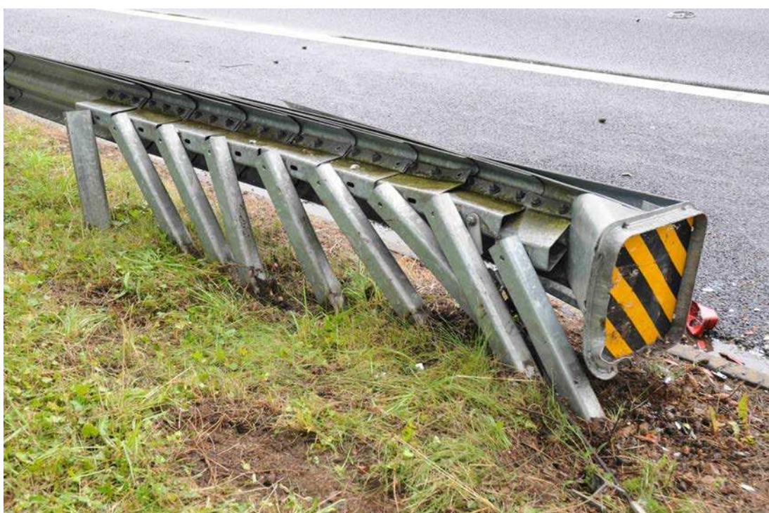
Figure 5.8(v): Compressed Roadside Barrier [GP]
