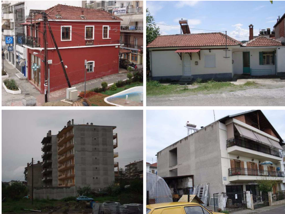
Fig. 1 Typical unreinforced masonry (top) and R/C (bottom) buildings in Grevena
