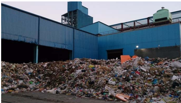
Figure 6: Waste at entrance to Rochem Power Plant
