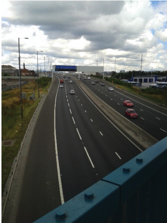
FIGURE 22 M74 extension passing beneath an existing street in Govanhill. Photograph © study participant and reproduced with permission.
