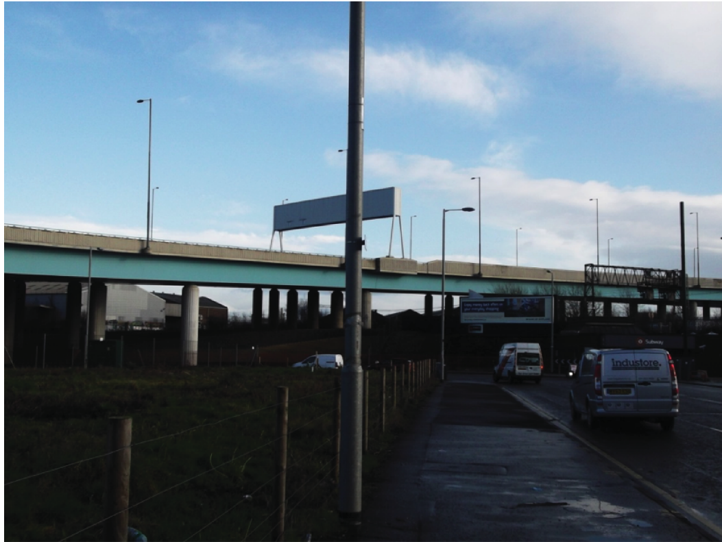
FIGURE 6 M74 extension crossing the Tradeston area on a viaduct. Photograph © Amy Nimegeer and reproduced with permission.
