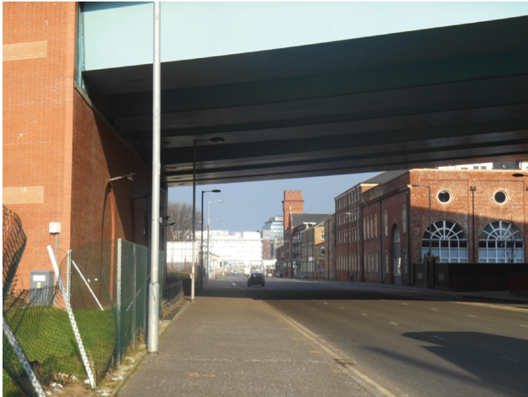
FIGURE 7 M74 extension crossing the Eglinton area on a viaduct. Photograph © Amy Nimegeer and reproduced with permission.
