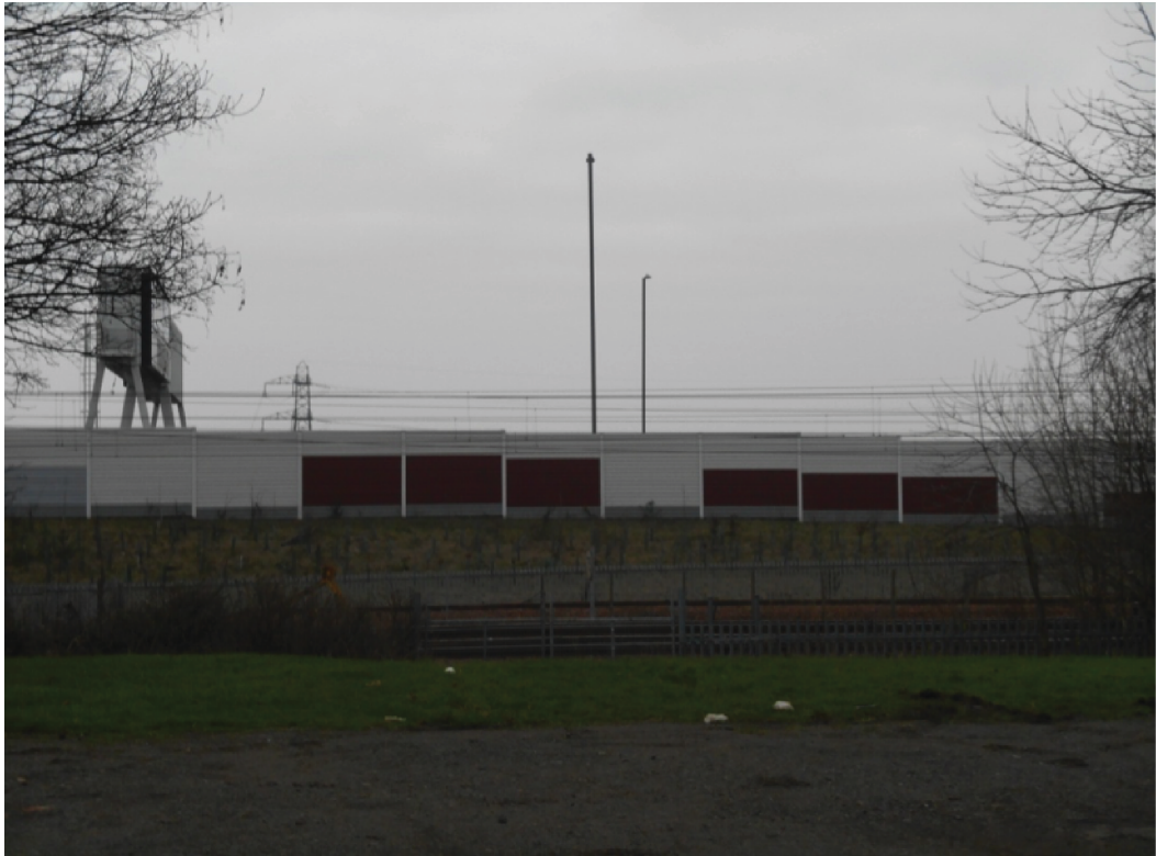
FIGURE 8 Noise barriers along the M74 extension at Rutherglen. Photograph © Amy Nimegeer and reproduced with permission.
