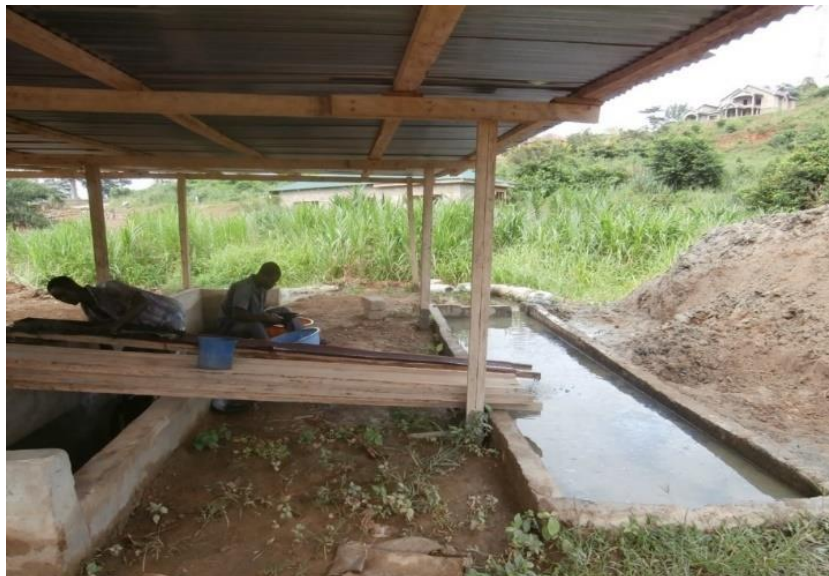
Figure 8.6 Sedimentation and tailing sump at an ASGM processing station.
