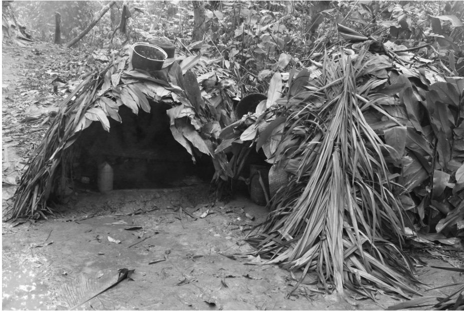
Figure 2-9: Two newly-made Mbendjele huts. The huts are made of flexible branches and Phrynium leaves.
