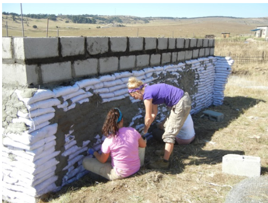
Figure 12: Students Applying Stucco
