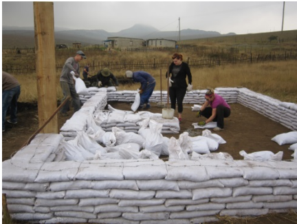
Figure 17: Building the Walls
