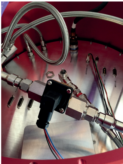
(a) Flow sensor mounted between the sealing plate feedthrough and the backflow umbilical shoe.
