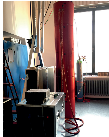
(b) Setup for flow measurement of the laser system cooling circuit. The chiller case shown in the front, with the sensor display on top. In the back the assembled payload with attached water umbilicals.
