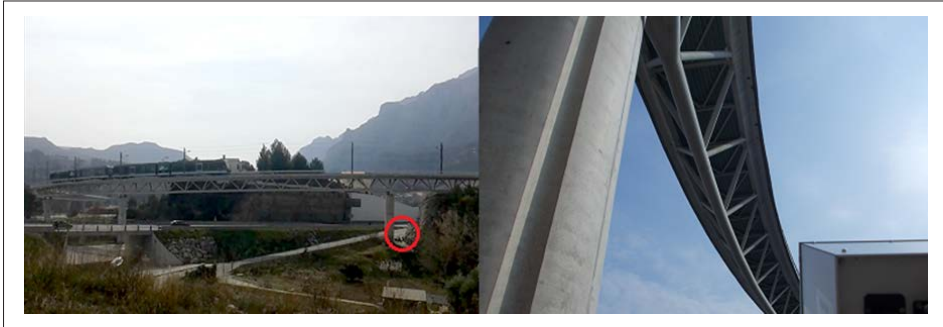
Figure 11 - Railway bridge measurement scenario. The red circle indicates the radar location.
