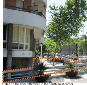
Detail on the level difference in the South West corner
