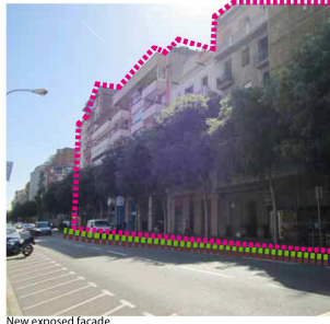
New exposed facade
