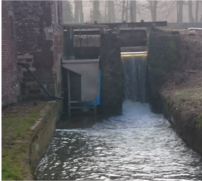
Figure 1.5: On-site Klerbeck plant
