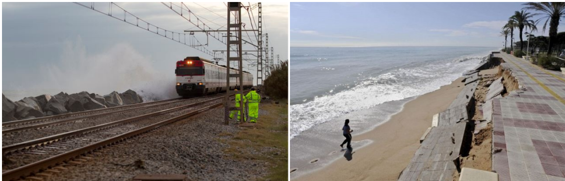
Figure 2.2: Train hit by waves in a railway located along the coast line (left) and damages in a promenade after a storm event (right) on the Catalan coast.
