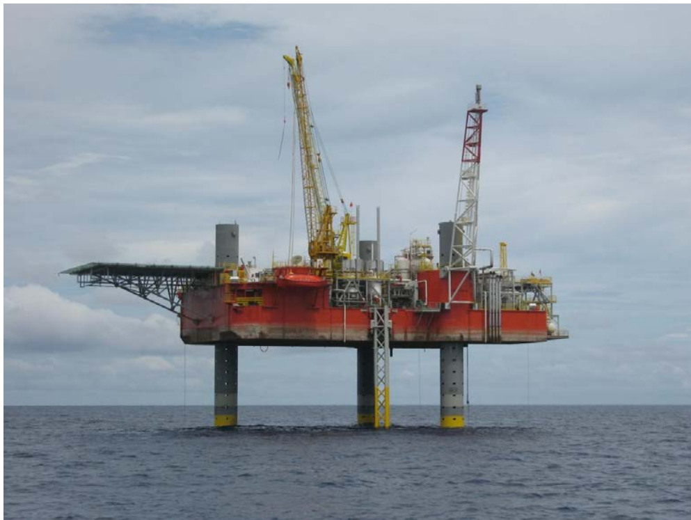
Figure 27: Platform CENDOR MOPU in place (from http://www.sediabena.com/oil-gas.html ). 40 men live there.
