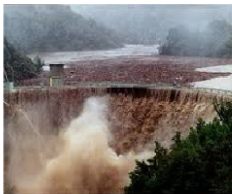
Figure 1.1: Overtopping in a concrete dam. Image taken from [18].
