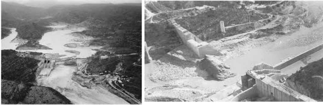
Figure 1.2: Images of Tous dam after the overtopping of October, 1982. Images taken from [1].
