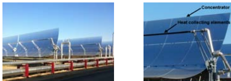
Image 2. Concentrator and heat collecting elements.
