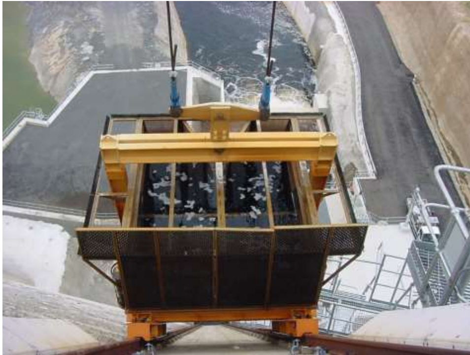
Figure 7 Fish elevator
