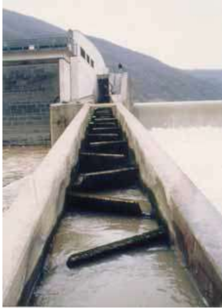
Figure 5 Rhomboid pool fish-pass
