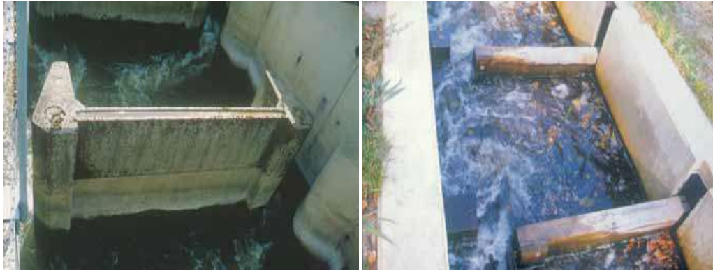
Figure 8 Vertical slot fish-passes (a) with two slots and guiding baffles (b) with one slot without guiding baffles
